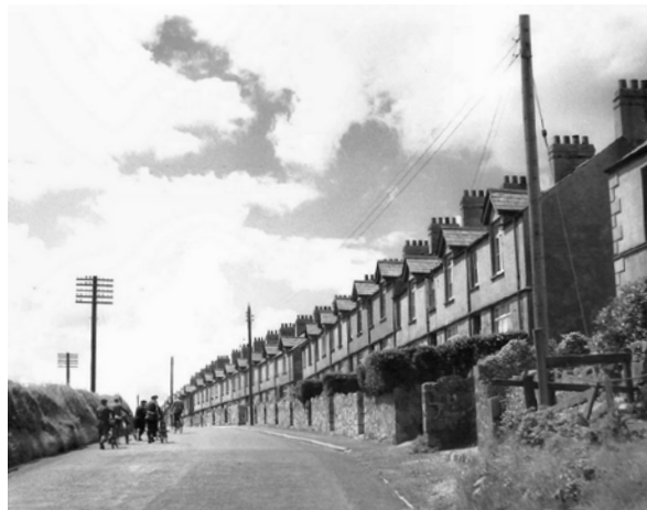
Figure 13: Foxhole, company houses, Main Street (CCHS 45746).
