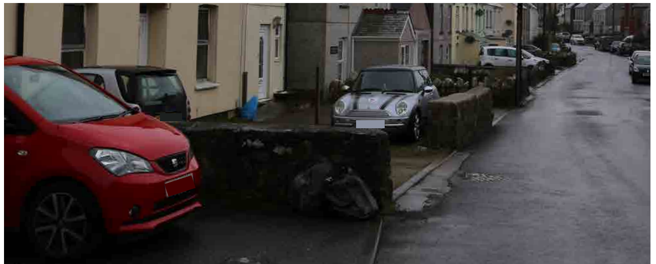
Figure 24: - Erosion of boundaries and front gardens.
