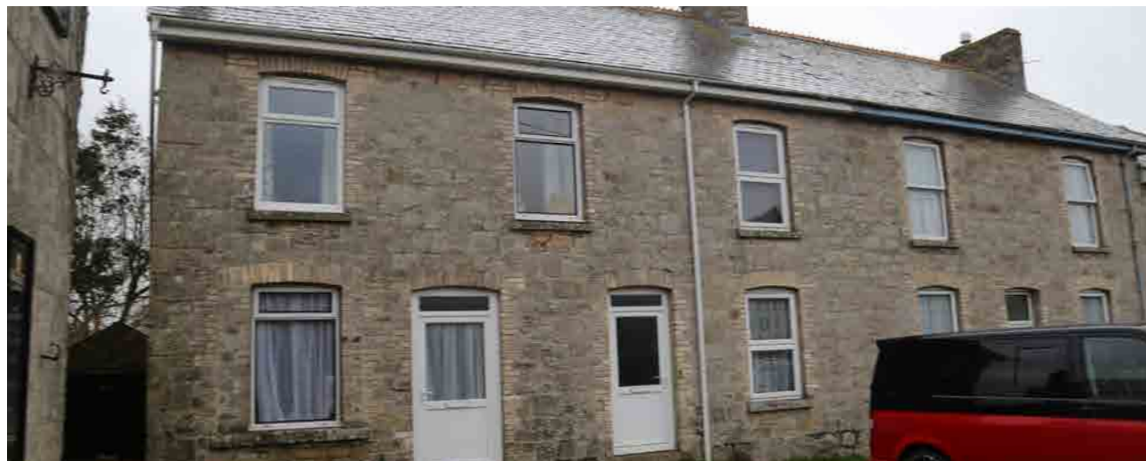
Figure 35: - Stone faced terrace with brick detail at lintel, window surround and door opening.
