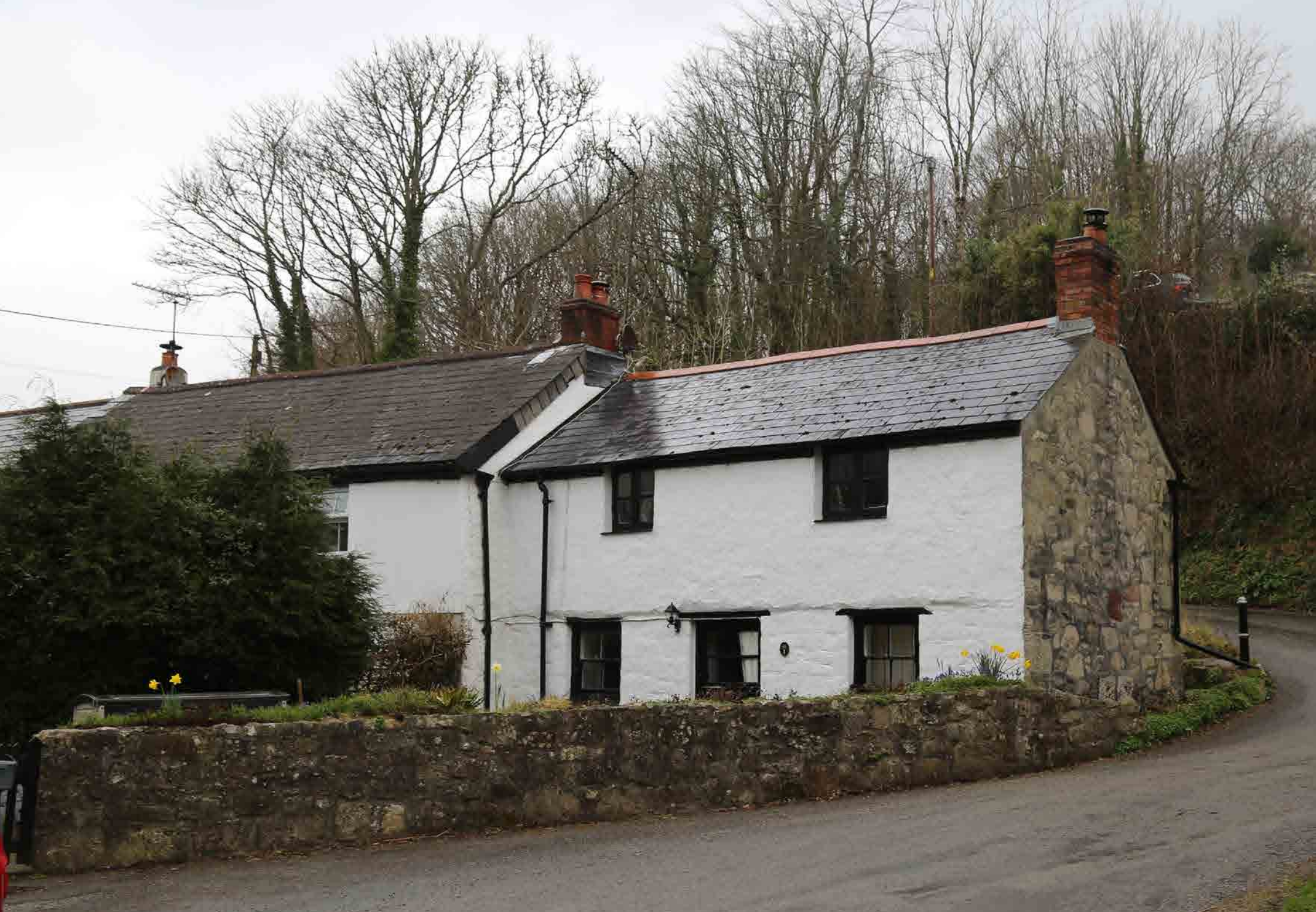
Figure 112: - Vernacular materials. Boundary is an extension of the property.
