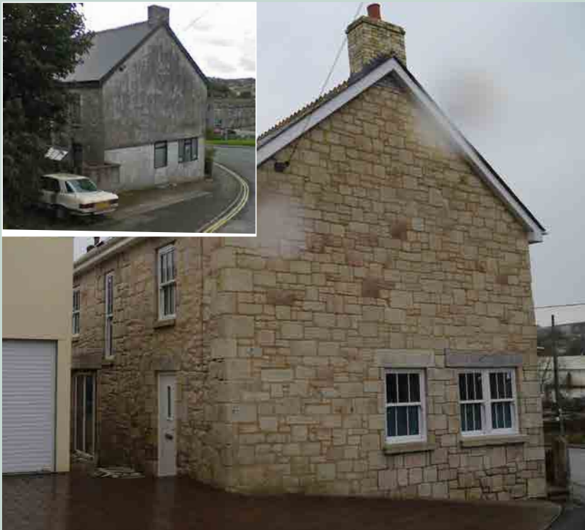
Figure 115: - Full renovation with stonework reinstated.
