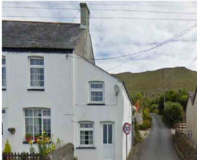
Figure 50: - Property directly beside road access.
