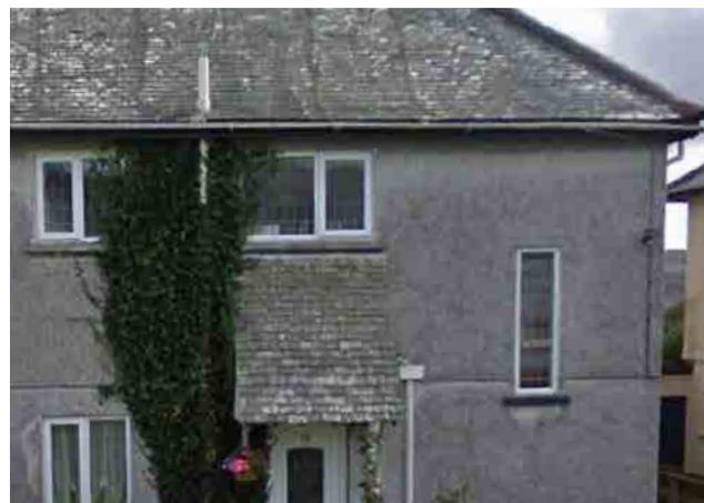
Figure 77: - Steeply pitched porch roof with diminishing slate courses.
