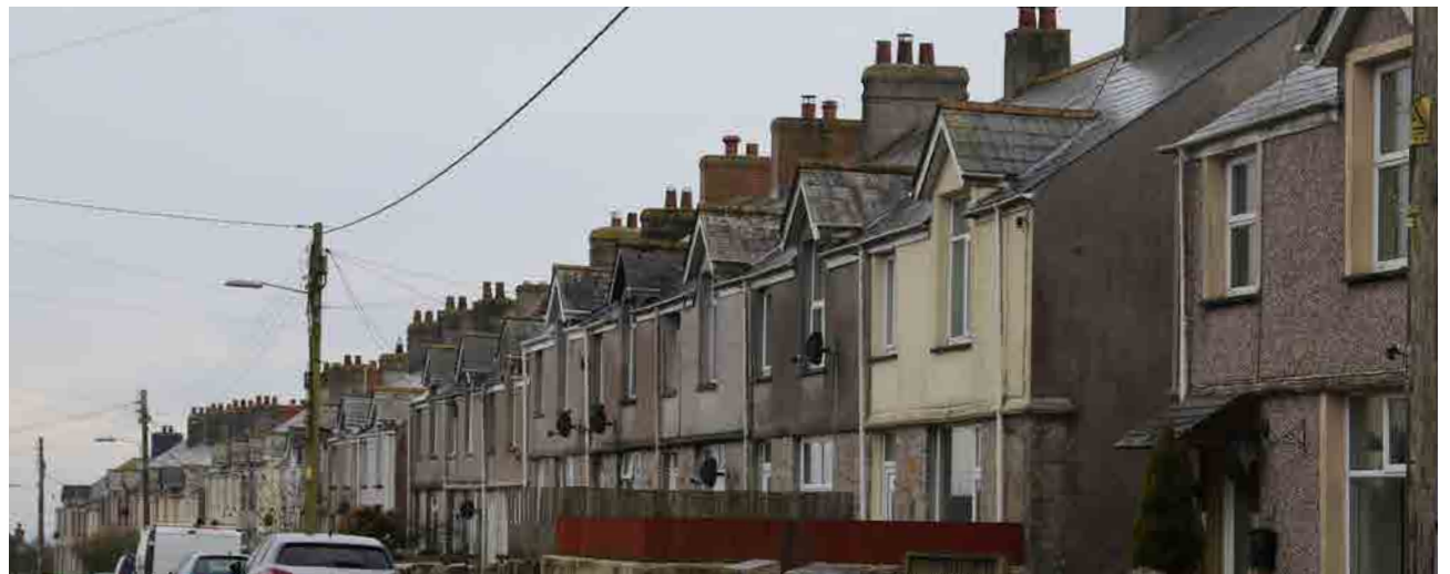
Figure 64: - Uniform terraces, with pitched dormer detail, creates distinctive rhythm to the front elevations.
