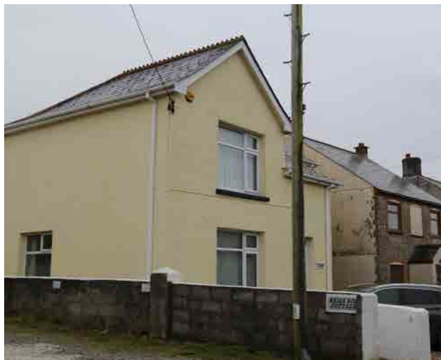
Figure 63: - Simple fenestration, large openings.
