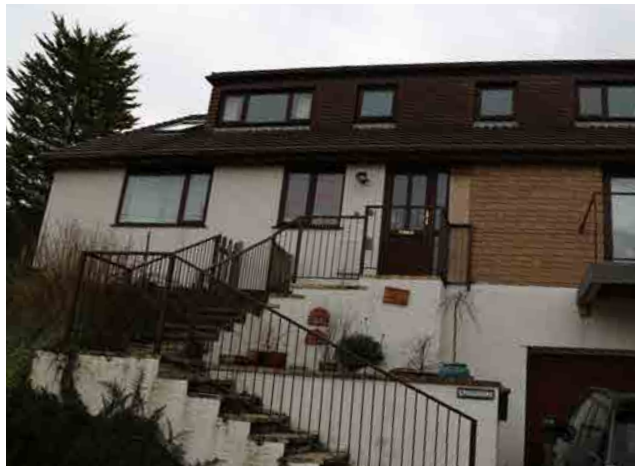
Figure 44: - Modern property with stepped access, concrete.
