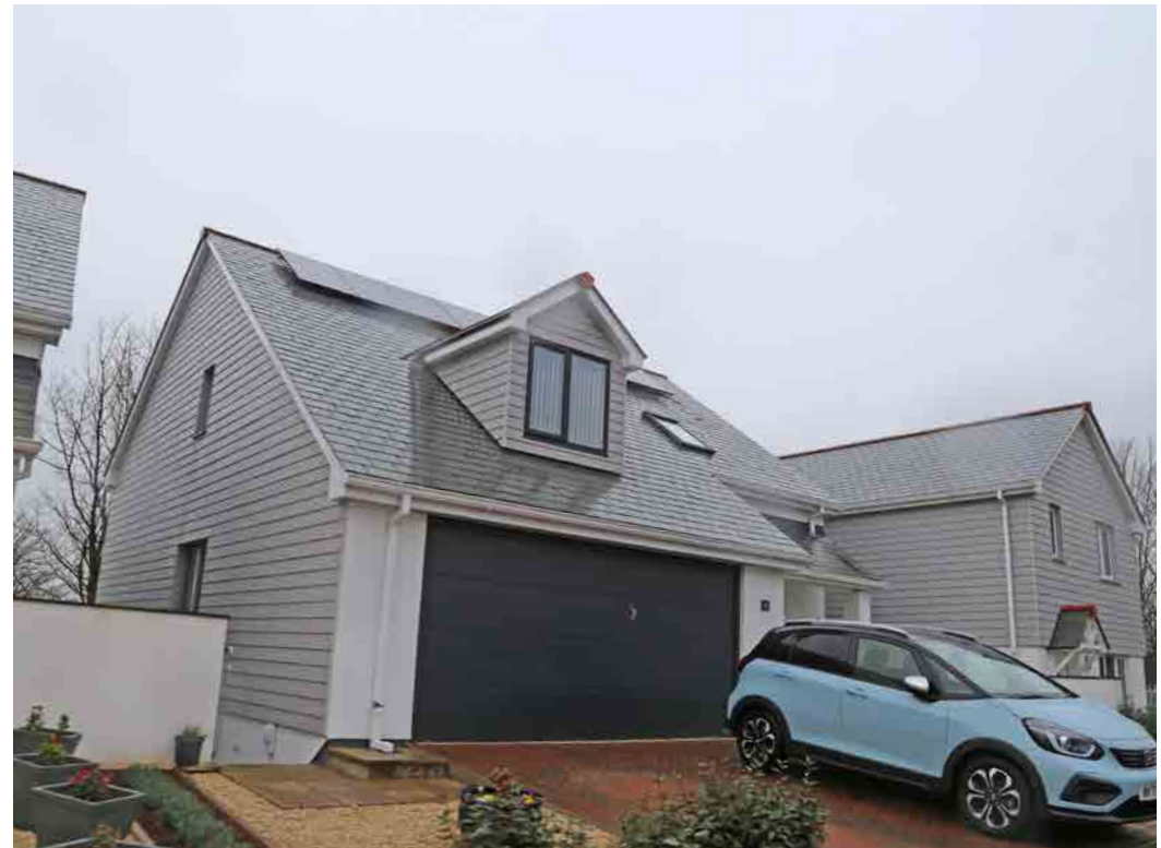
Figure 105: - Good example of an architectural response to topography as property steps down at the rear.
