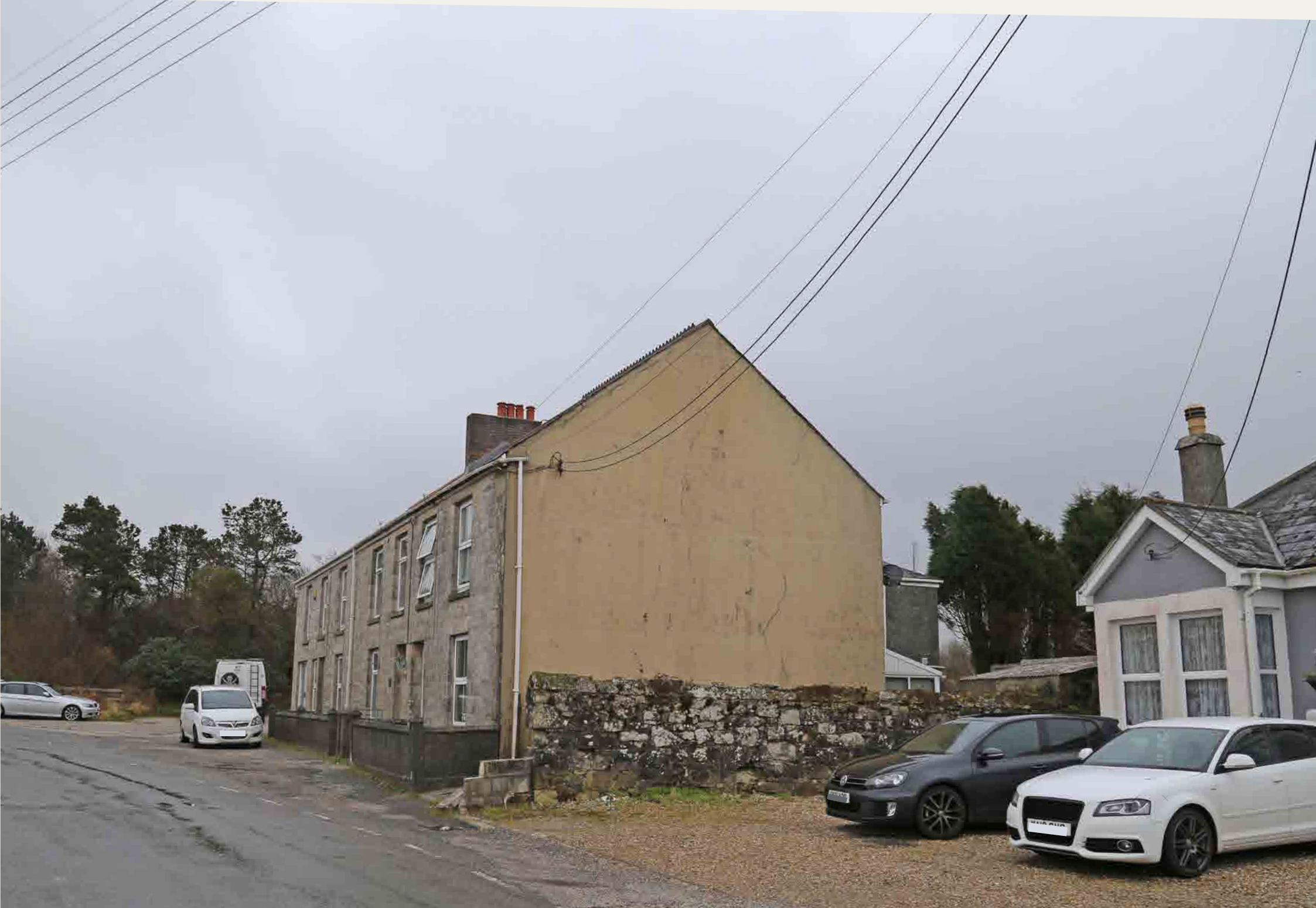
Figure 81: - Short terrace, stone construction with rendered gable.
