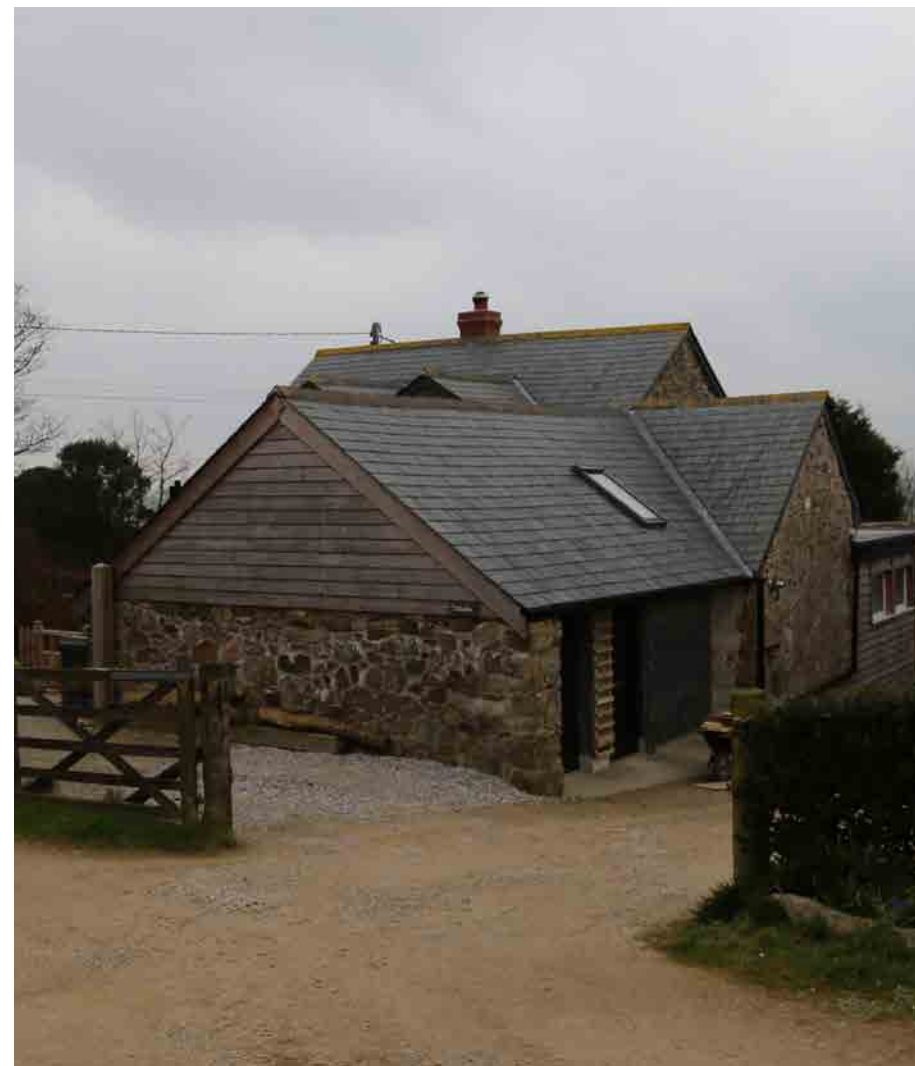
Figure 114: - Barn/outbuildings renovated and re-purposed as characterful addition to principal dwelling.
