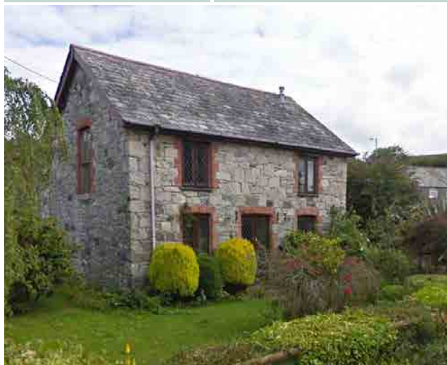
Figure 47: - Stone built, contrasting brick at openings.
