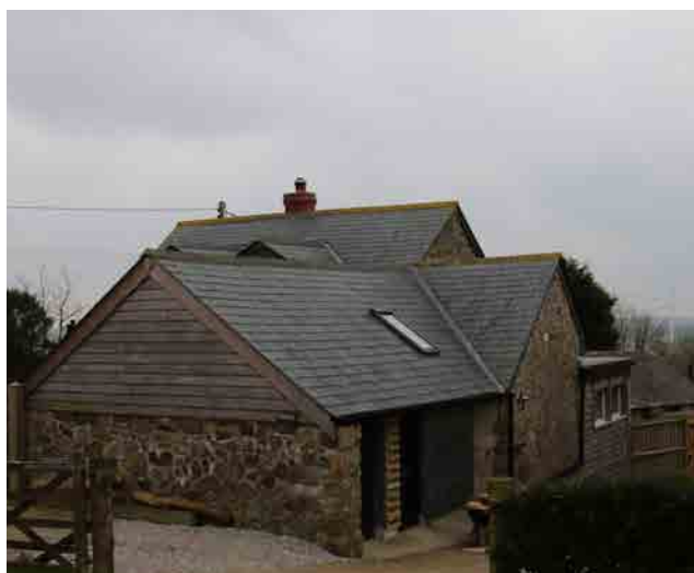
Figure 87: - Modernised farm building. Stone with timber cladding.
