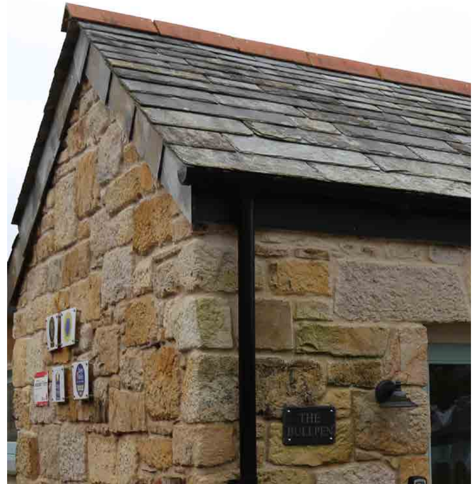
Figure 106: - Example of diminishing course slate roof and stone construction.
