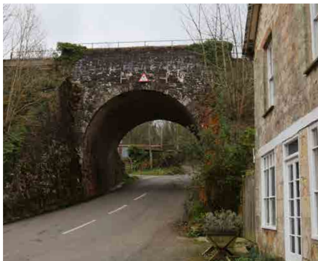
Figure 39: - Village railway bridge gateway.
