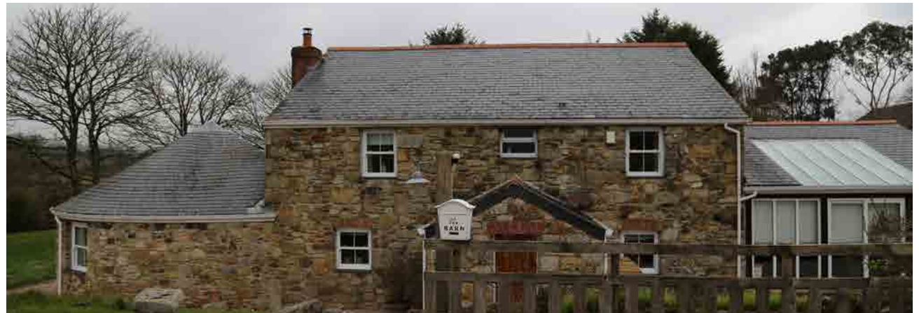
Figure 93: - Conical extension finished in slate with scalloped leadwork.
