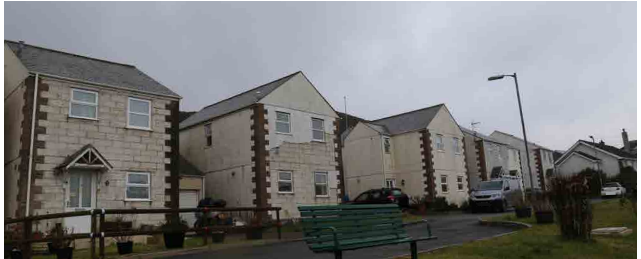
Figure 83: - Carn Bargas construction defect.
