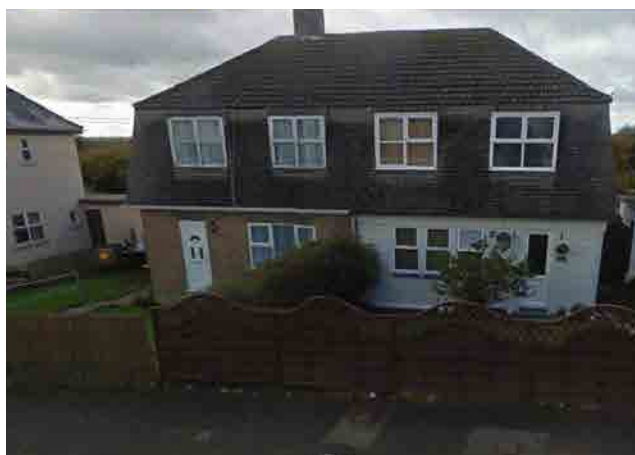
Figure 36: - Original Cornish unit beside upgraded version (brick).
