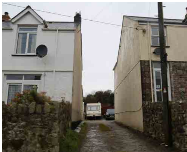
Figure 71: - Terraces in blocks punctuated by rear access lanes.
