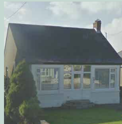
Figure 127: - Subtle porch enclosure.
