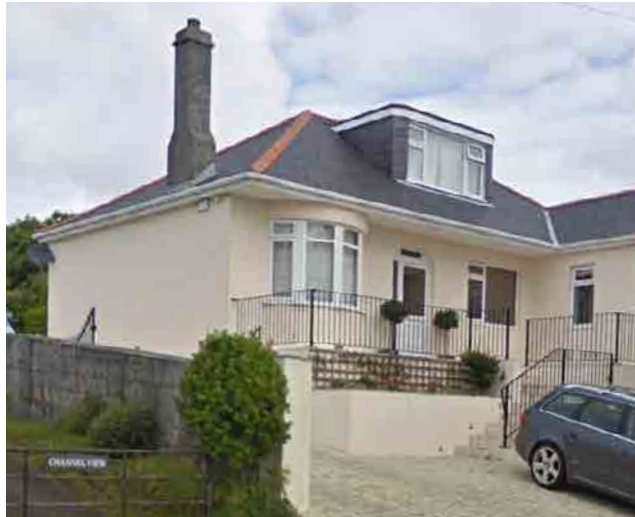
Figure 58: - Stepped access to bungalow, roof dormer.
