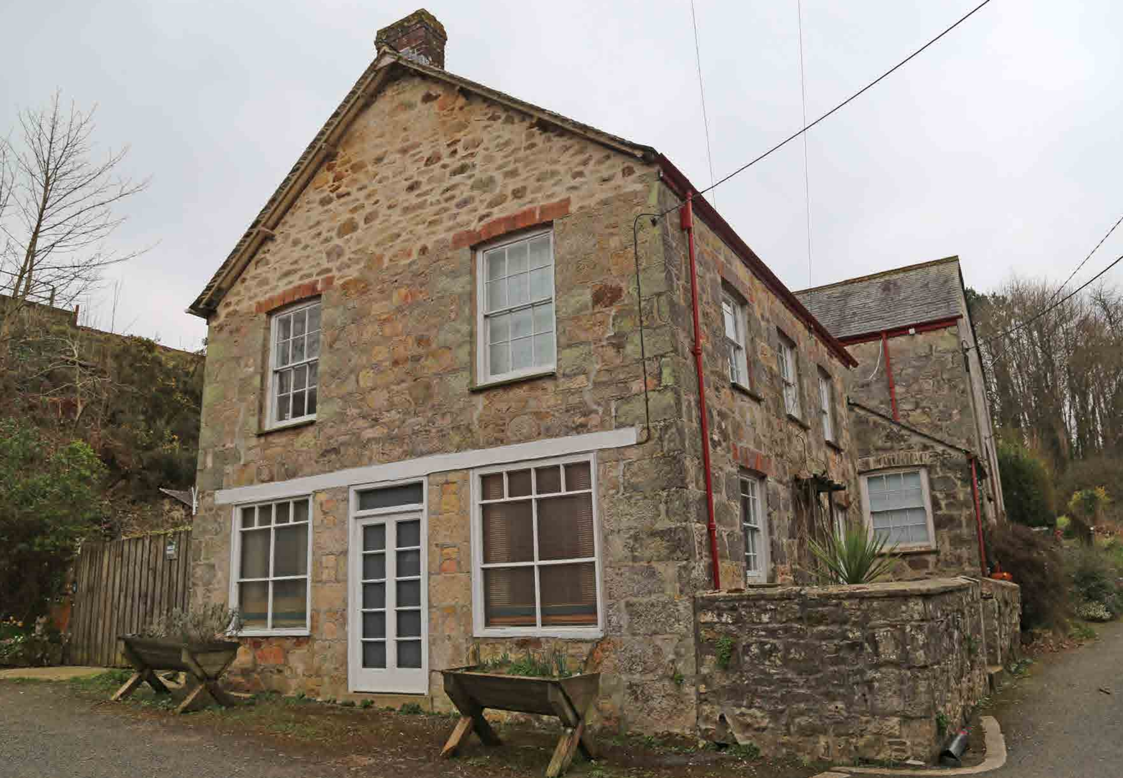
Figure 95: - Coombe property stonework character
