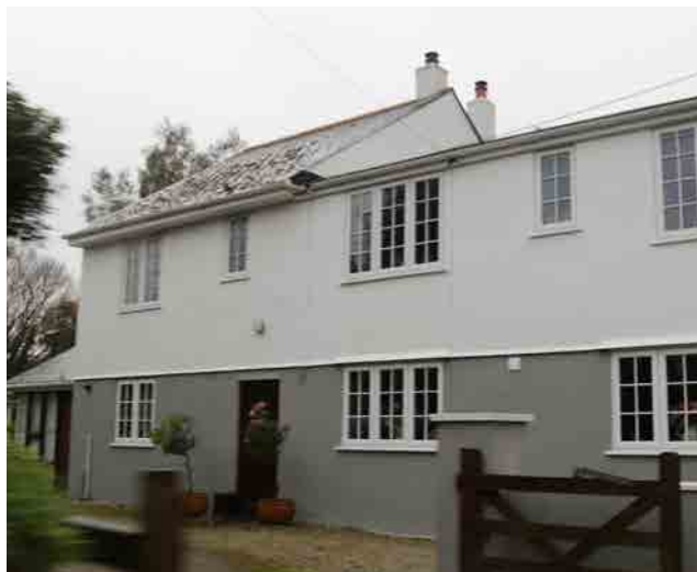
Figure 55: - Roof variation, smooth finish rendered façades.
