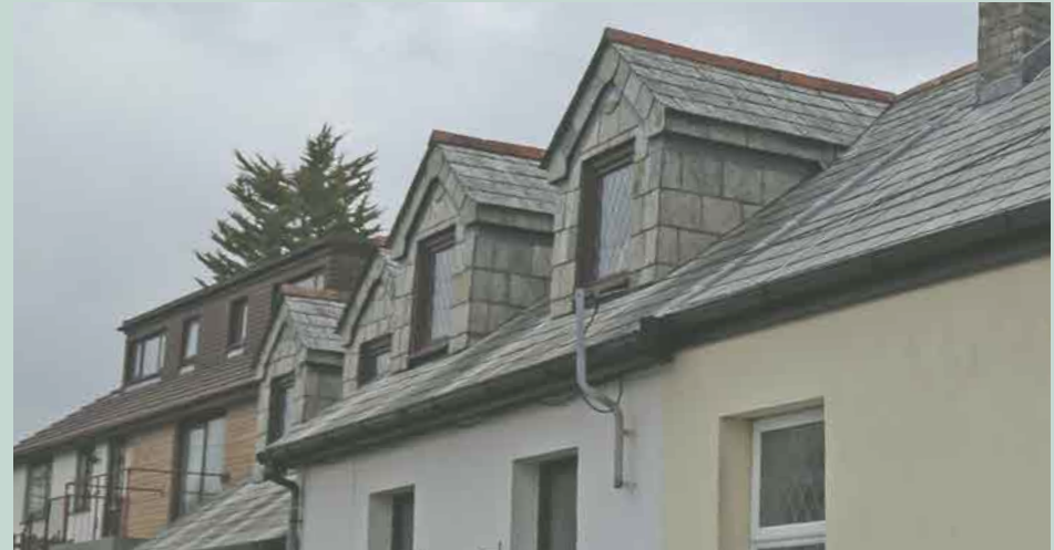
Figure 116: - Well detailed pitched dormer in slate hanging.
