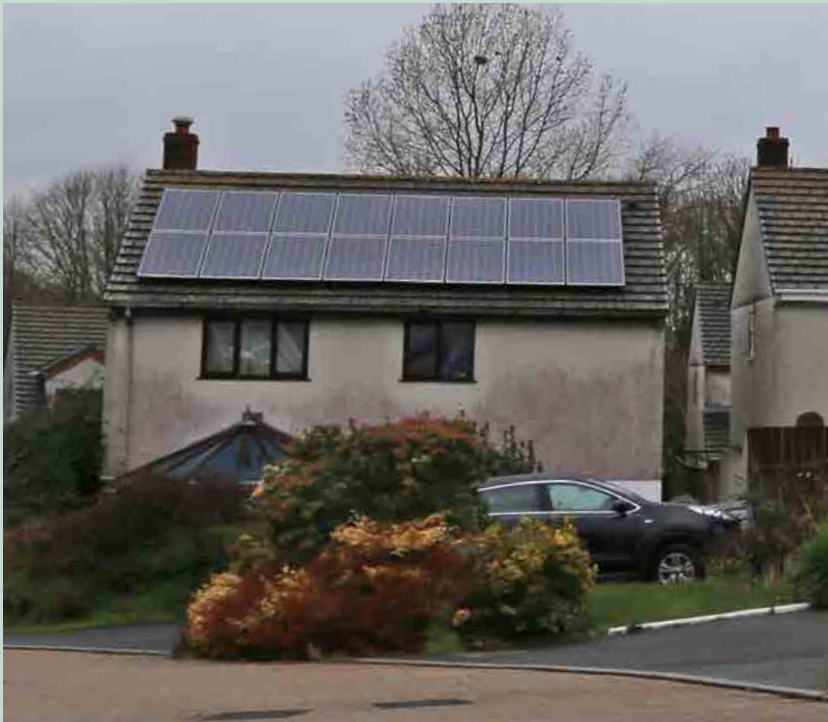
Figure 125: - Renewable energy PV array.
