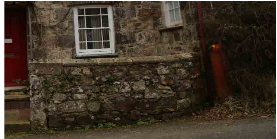
Figure 123: - LPG connections on-street, presents safety risk.
