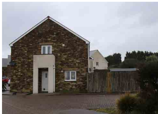
Figure 69: - Unusual porch/balcony space.
