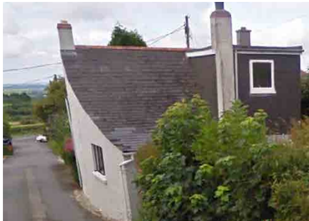
Figure 60: - Primitive rear extension, flat roof dormer.
